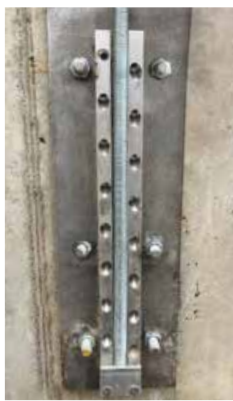
MEGANT® concrete connection.
