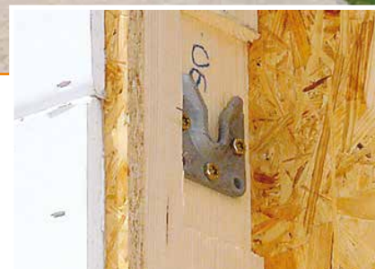
Installation example: wall connection.
