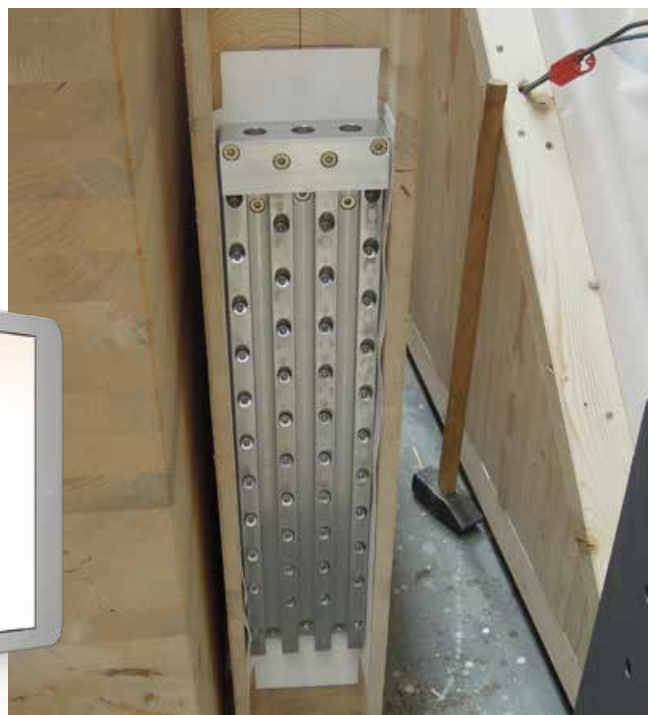
MEGANT® with fire protection Firestrip Interdense Type 15 for protecting the connector from heat in case of fire.
