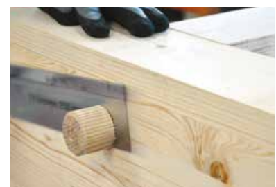
Cut and sand the excess part
