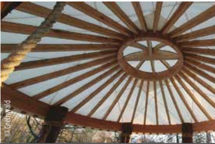
Inclined rafter connections attached to the top of the dome with T-JOINT.
