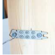
Install the locking clip
