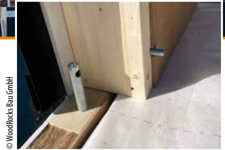
Detail : Pipe System - wall to wall joint.
