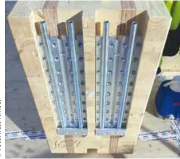
Three-sided concealed assembly by milling into the secondary beam. MEGANT® is fixed to the main beam with no need for milling.
