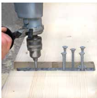
Screw on RICON® S on Header
