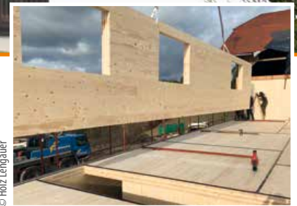
Installation example: CLT walls installation.
