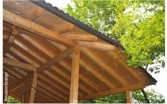
Carport without brace.
