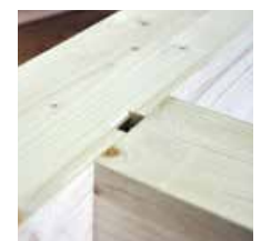
Secured connection using a locking clip
