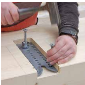
Position the plate and the screws
