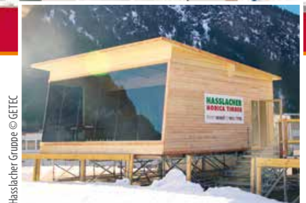
Installation example: ORF-Studio, Oberstdorf, DE.
