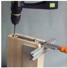
Pre-drill with drilling-jig
